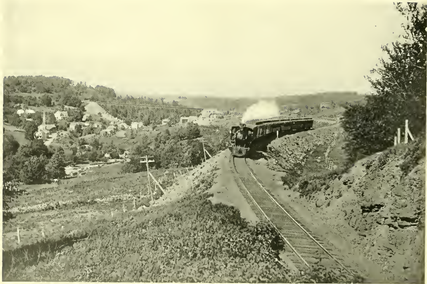
Ferndale — showing Railroad Bridge
